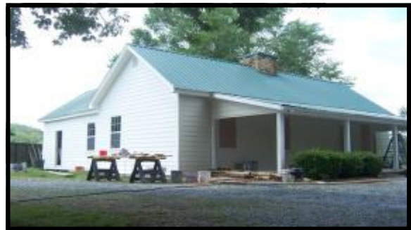
Our new welcome center finished in July.
