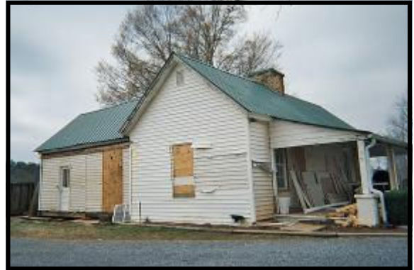
Demolition under way at the old homestead.
