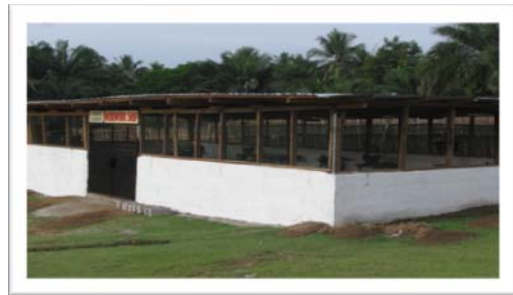
External view of the Wood work shop – BFC
