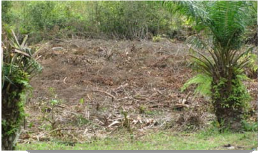
Brushing the swamp to prepare the Agr. Site
