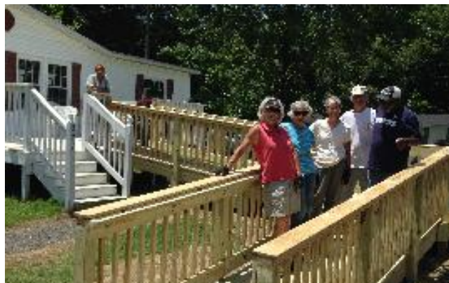
Bruton Builders, in conjunction with Housing Partnerships constructed this ramp for a happy, Toano homeowner.
