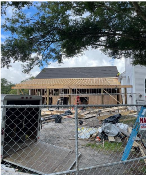
Framing covered porch roof in process
