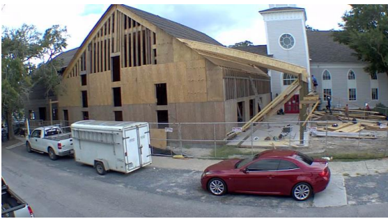
Framing covered porch roof in process
