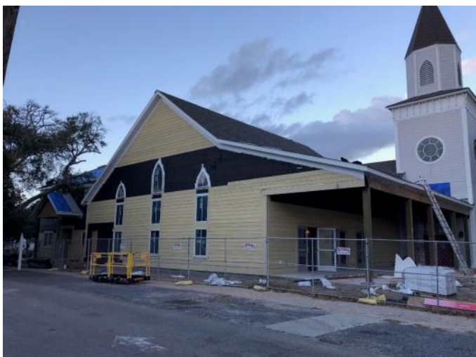
Shingle Install Completed
