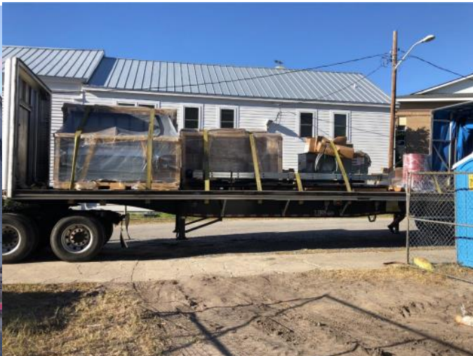
Elevator Delivered and install to begin
