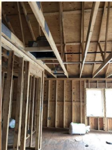
Heating and Air rough ins in progress
