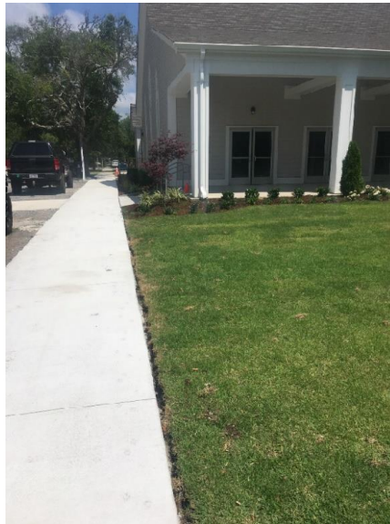
New Sidewalk installed
