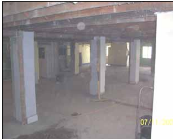
"Lower level 'opened up'! Note how spacious the area has become."
