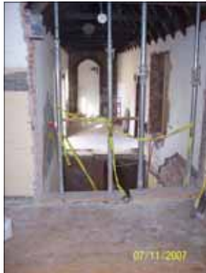
"Breezeway just prior to demolition"
