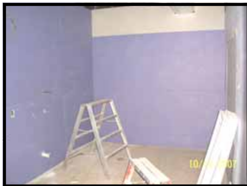
New restroom in Cary Lounge area.
