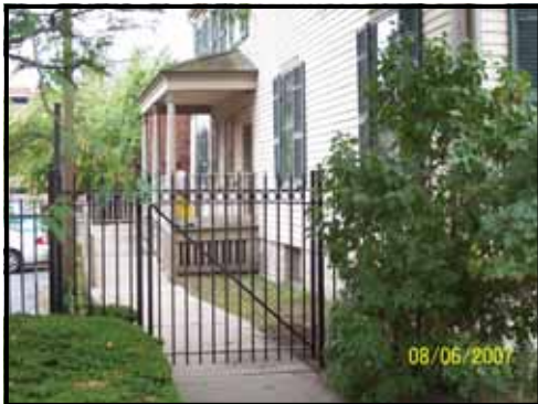
Ramp entrance to Sibley House.
