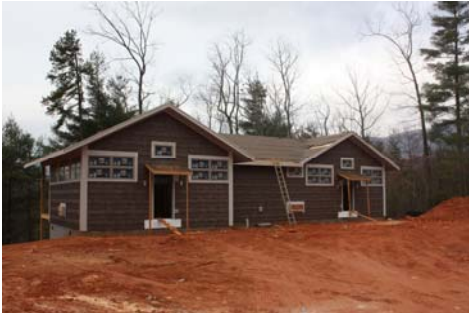
New cabin under construction
