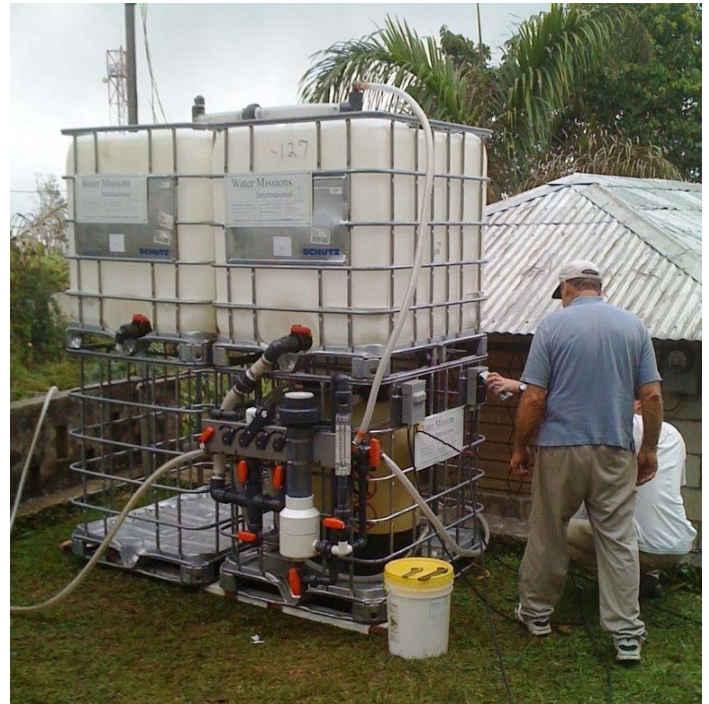
Water Missions International workers assembling a water purification unit in Haiti
