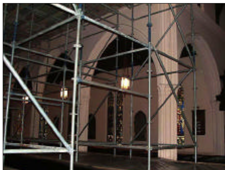
Scaffolding inside Cathedral
