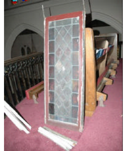
1846 window South and North Towers
