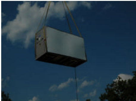
Installation of one of two chillers
