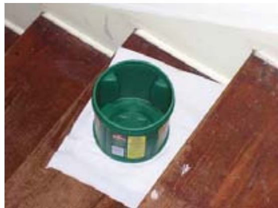
We need a better solution for a leaky roof!
