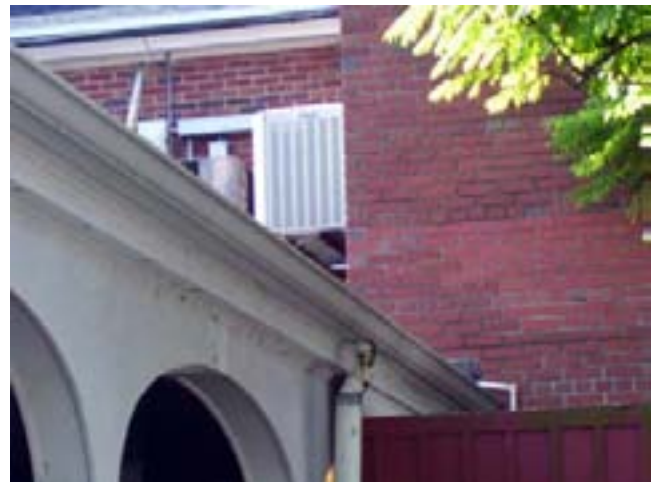
Roof Unit above the Office Building
